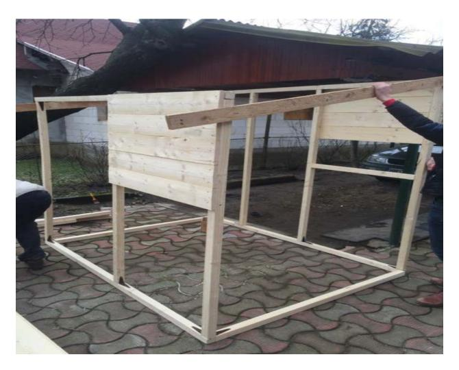
Step #6 - Nailing wood boards on the exterior of the cage
